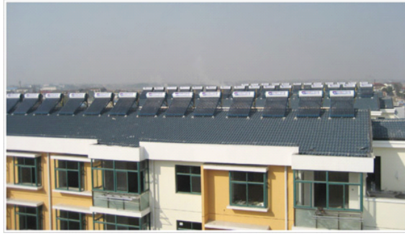
Figure 5 Solar-absorbent materials to heat bathwater
